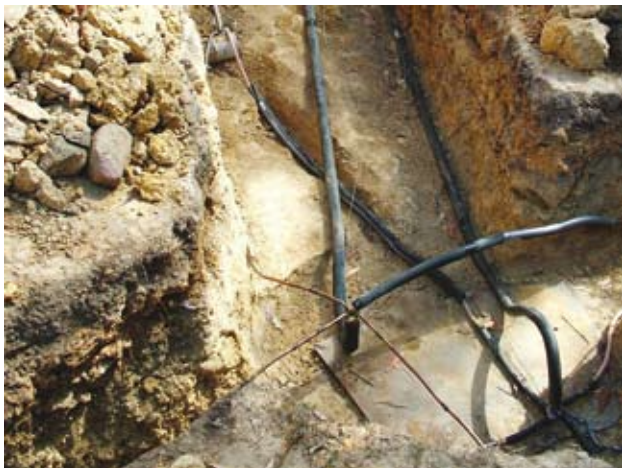
A prototype geothermal cooling system is being trialled at CSIRO's Marsfield site. Photo Credit: Grant Hampson, CSIRO.
