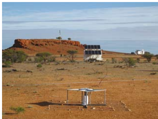
The EDGES antenna (in the foreground) at the MRO. Under the antenna, in a white protective envelope, is an analog receiver chain with internal comparison-switched calibration noise sources. The cable leads back 70 metres to the CSIRO trailer, which houses a direct-sample digitiser. Photo Credit: Judd Bowman, Caltech.
