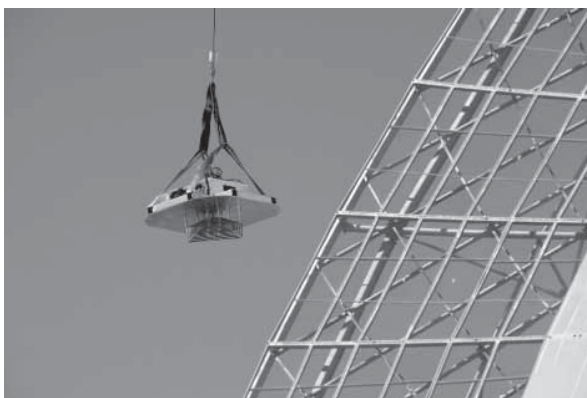
Installation of a 300 – 900-MHz receiver on the Parkes 64-m radio telescope. The wideband feed is based on the Eleven Feed, designed by Per-Simon Kildal of Chalmers University, Sweden.
