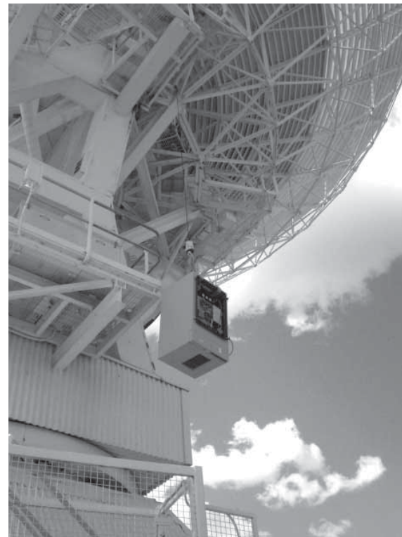
A new CABB antenna rack being lifted into an antenna for fitting.
