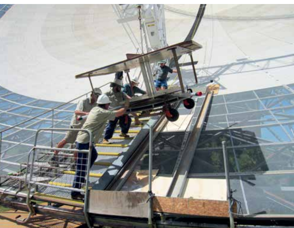
Installation of the 'Erickson' feed at Parkes during the February shutdown.
