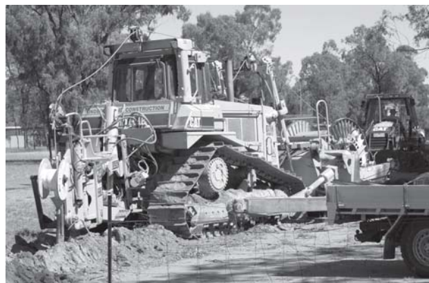
Figure 2: A cable-laying machine burying the broadband fibre near the central area of the Narrabri Observatory.
