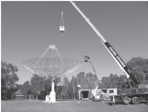
The THEA tile being mounted on the eastern New Technology Demonstrator antenna.
