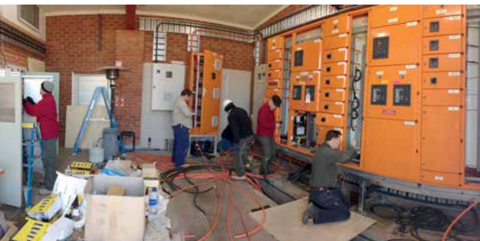
Installing the new electrical switchboard at Parkes
