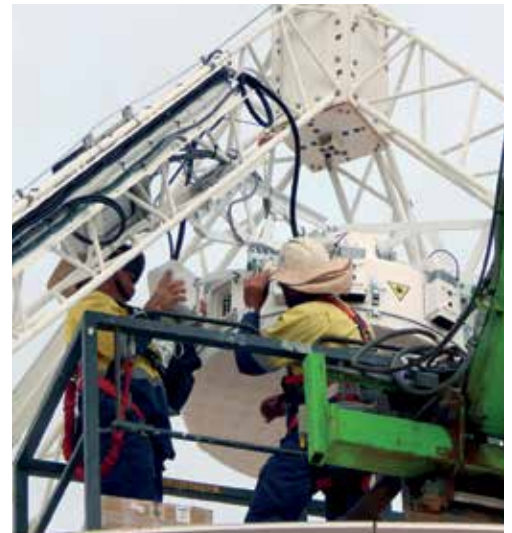
The Mk II prototype phased-array feed being installed onto ASKAP Antenna 29.
