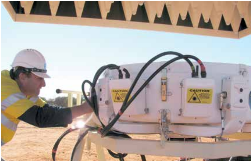
The set-up used for the 'hot' observation of an absorber box during 'on ground' tests of the prototype Mk II PAF at the MRO.
