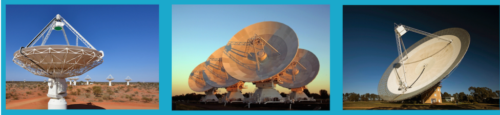
Figure 1. ATNF radio telescopes. — From left to right: ASKAP (36 × 12-m dishes equipped with wide-field Phased-Array Feeds (PAFs); 6-km diameter), ATCA (6 × 22-m dishes; 6-km diameter) and the 64-m Parkes Telescope as featured in the ATNF Daily Astronomy Picture (ADAP: www.atnf.csiro.au/ATNF-DailyImage/ created by B. S. Koribalski).
