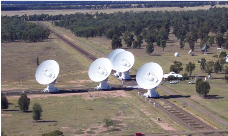
Figure 1.1: An aerial photo showing five ATNF Compact Array antennas, in a compact millimetre-wave configuration, with new solid panels in place. The North/South spur can be seen extending from the main line towards the left of the photograph.
