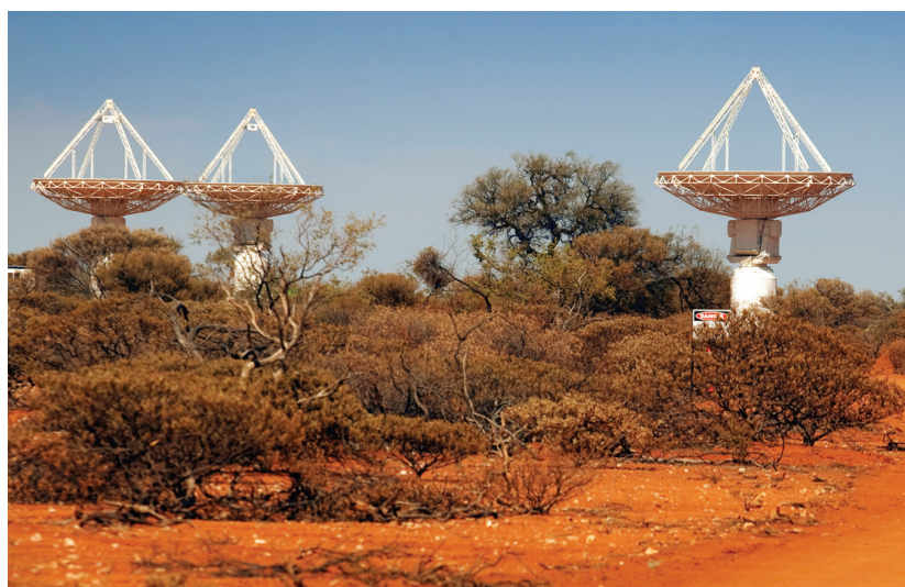
> Three newly constructed CSIRO ASKAP antennas pictured at the Murchison Radio-astronomy Observatory in Western Australia, October 2010.
