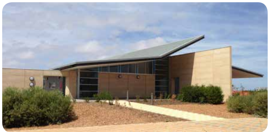
CSIRO's MRO Support Facility in Geraldton.
