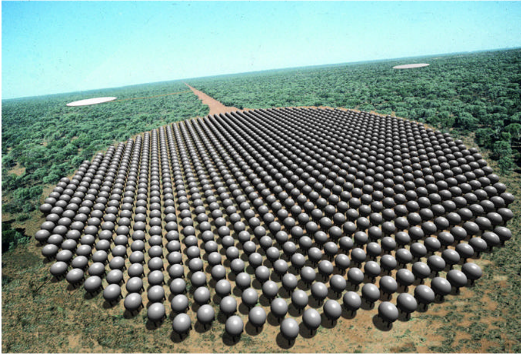
Figure 2. Artist's impression of an SKA station composed of 400 Luneburg Lens antennas, each 5 m in diameter. The station has the same collecting area as a 100 m diameter dish, but can form many simultaneous, widely-spaced, beams on the sky. More than 100 such stations would be required for the SKA.
