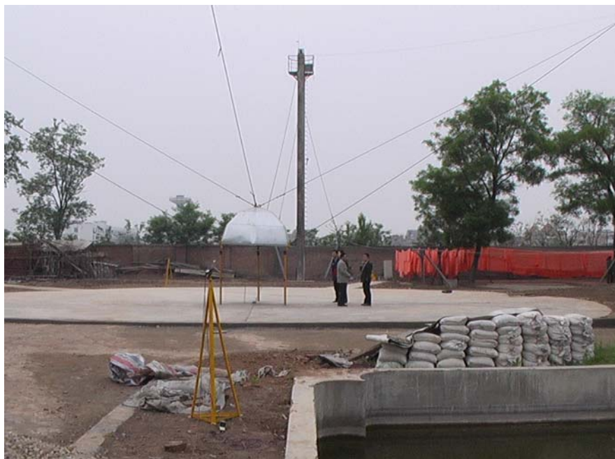
Fig.12-6 A 50\text{ m} \times 50\text{ m} \times 15\text{ m} model of the cable-support structure developed
