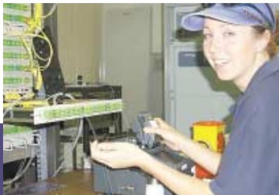
Leigh Panton, an apprentice with the ATNF Narrabri electronics group, splicing fibres at a patch panel in the screened room
