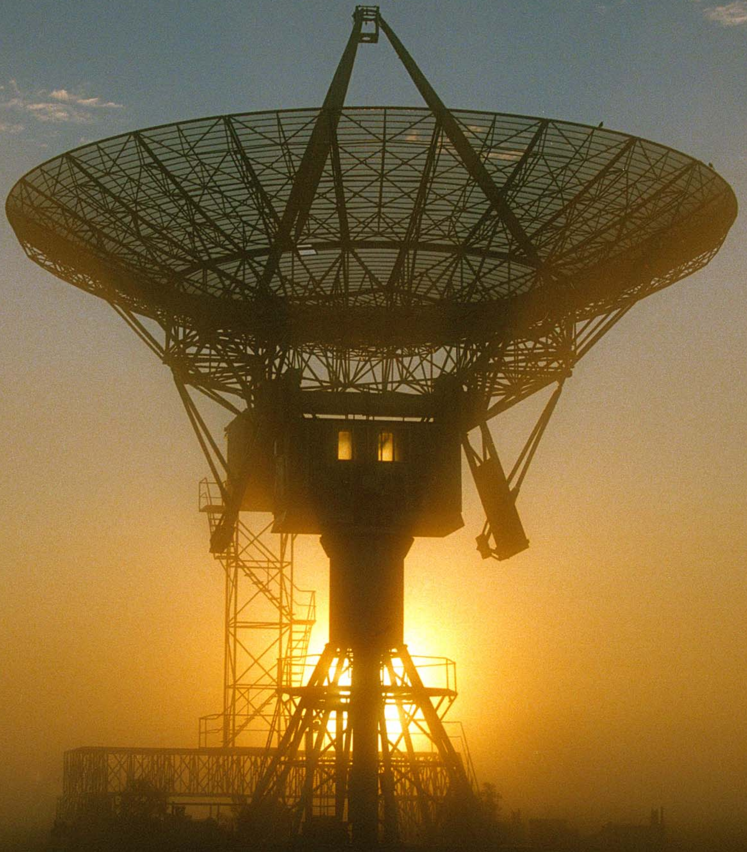
The Kennedy 18-m antenna at Parkes was originally used in Australia at the Fleurs radio astronomy site. It was transferred to the Parkes site in 1963.
