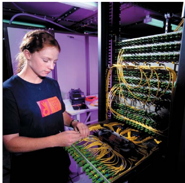
Alison Ryan working on optical fibre connections for the local oscillator distribution network at the Compact Array.
