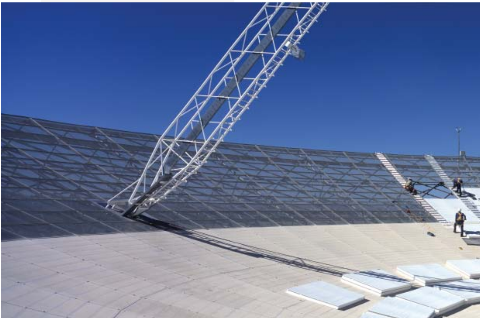
Work in progress to replace some of the panels on the surface of the Parkes radio telescope, in preparation for the NASA Mars tracking program. Photo: © Tim Ruckley
