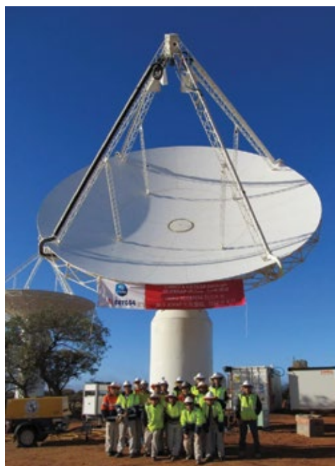
Members of the CETC54 and ASKAP teams celebrate assembly of all 36 ASKAP antennas in May 2012. Final site acceptance tests have since confirmed reflector accuracy better than ASKAP specification, meaning that the antennas will be able to operate at up to 20 GHz.
