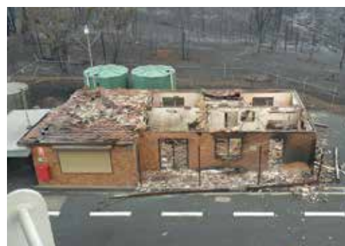
The bushfire destroyed the accommodation area of the Mopra control building, but the main control room (at left) was protected by its concrete structure and screening on the door and windows. Credit: Tim Wilson
