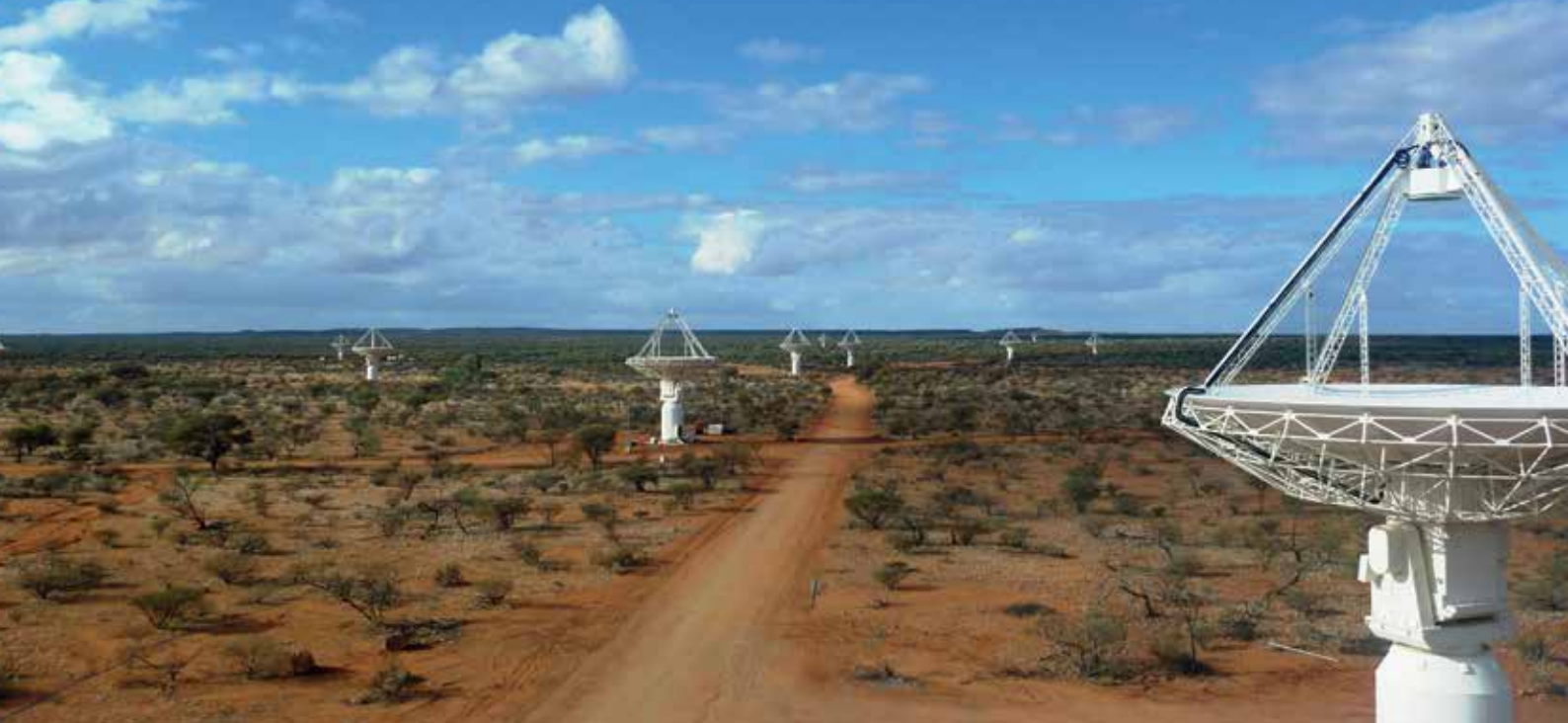
Six first-generation phased array feeds were installed on antennas of the Australian SKA Pathfinder this year, forming the Boolardy Engineering Test Array (BETA). Credit: Steve Barker
