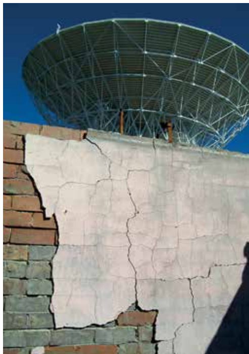
January's bushfire destroyed much of the control building at the Mopra site but left the antenna structure untouched. Credit: Tim Wilson
