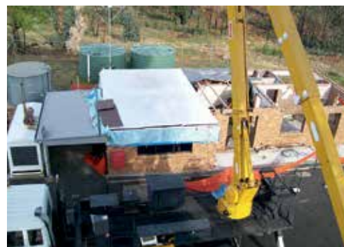
Repair work under way. Credit: Tim Wilson
