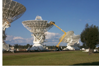
The Antenna Structure
