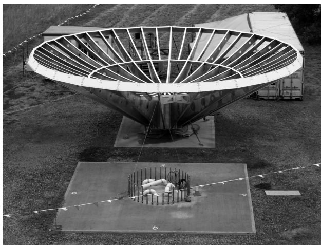
Reflector assembly on 18 January 2008 – awaiting installation of panels
