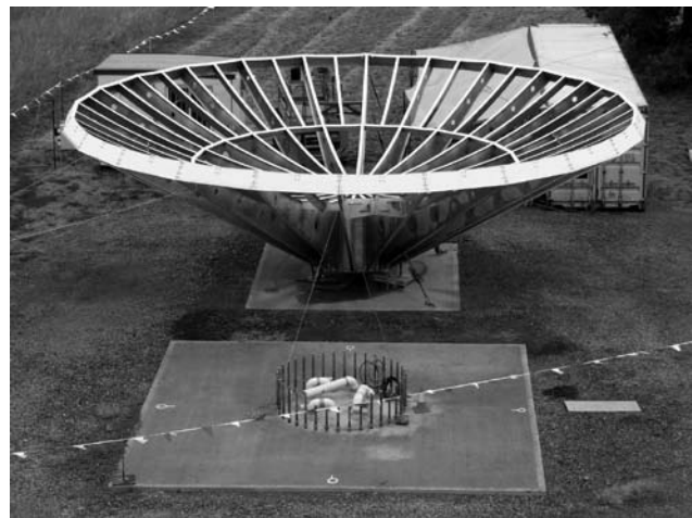
Reflector assembly on 18 January 2008 – awaiting installation of panels
