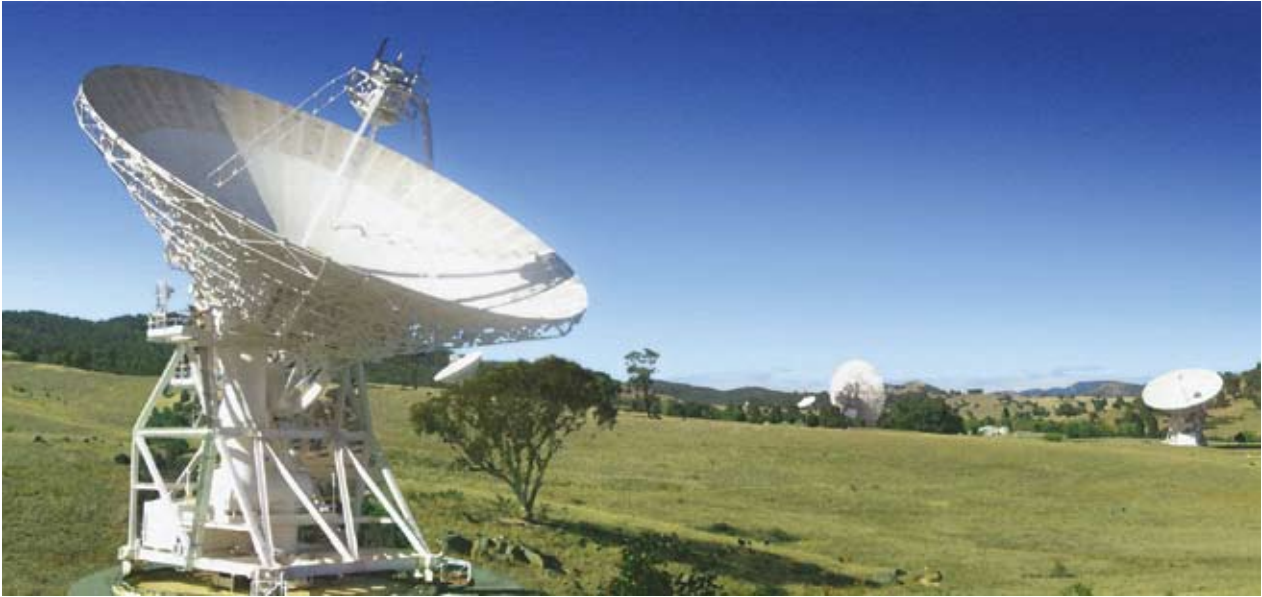
An artist's impression of the new DSS35, 34-metre Beam Wave Guide antenna to be constructed at the Canberra Deep Space Communications Complex, Tidbinbilla. Credit: CDSCC/NASA
