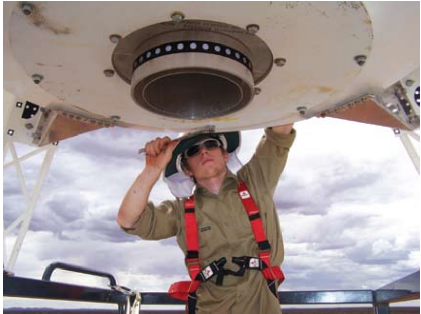
Ben Lauter from the main workshop tightening the last bolts, 17m in the air in the basket of the telehandler. Credit: R Forsyth, CSIRO
