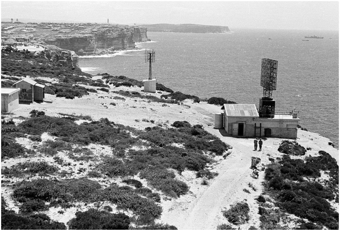
Figure 2: RPL field station, Army Reserve, Dover Heights; the Fortress Fire Command Post was in this reserve, 2.2 km south of the Macquarie Lighthouse and 2 km north of Bondi Beach. The location is 7 km east of the centre of Sydney. Date, 18 February 1943. This 200-MHz antenna, associated with the main blockhouse, was used for the solar radio astronomy sea-cliff observations on Australia Day, 1946. The view is to the north with North Head clearly visible. Note the ships possibly waiting for the submarine net at the entrance to Sydney harbour. (ATNF historical photographic archive B81-I)
