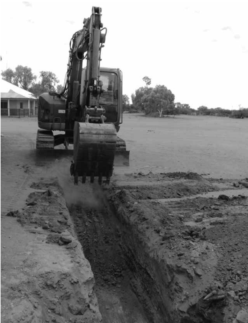
Trench digging underway near the Boolardy homestead. Credit: Barry Turner, CSIRO
