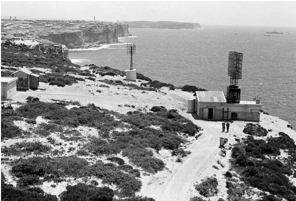
Figure 2: RPL field station, Army Reserve, Dover Heights; the Fortress Fire Command Post was in this reserve, 2.2 km south of the Macquarie Lighthouse and 2 km north of Bondi Beach. The location is 7 km east of the centre of Sydney. Date, 18 February 1943. This 200-MHz antenna, associated with the main blockhouse, was used for the solar radio astronomy sea-cliff observations on Australia Day, 1946. The view is to the north with North Head clearly visible. Note the ships possibly waiting for the submarine net at the entrance to Sydney harbour. (ATNF historical photographic archive B81-1)
