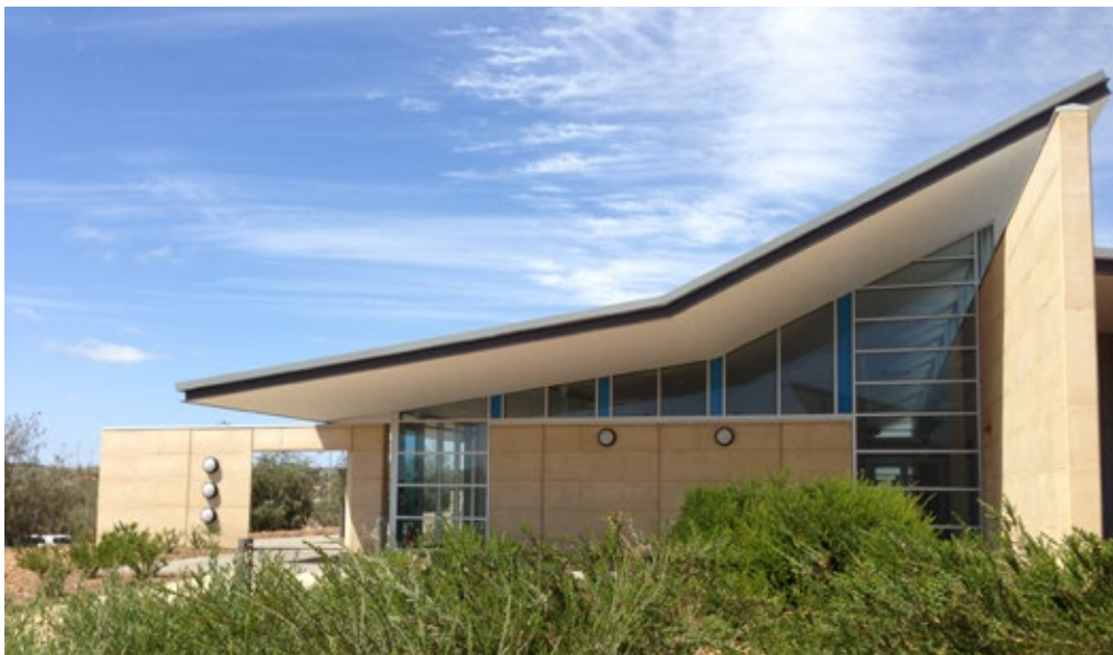
The new MRO Support Facility in Geraldton.
