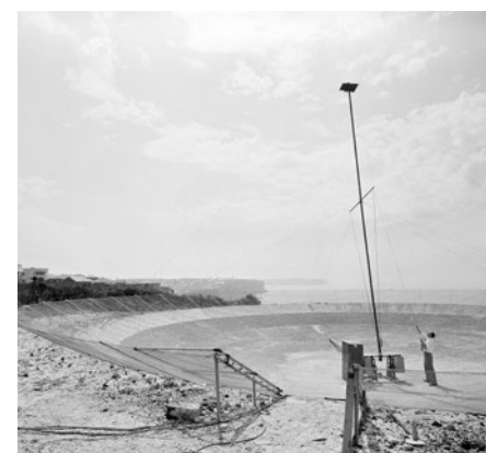
Radiophysics’ upgraded, 80-foot ‘hole-in-the-ground’ radio telescope at Dover Heights, Sydney. In this photograph, taken in 1953, Gordon Stanley is adjusting the position of the aerial mast.
