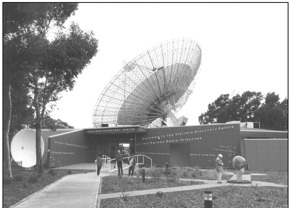
The Visitors Centre at the Parkes Observatory
