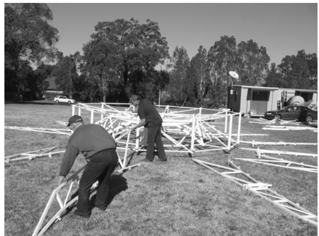
Figure 2: Early meccano training comes into good use in reconstruction of the NTD antenna! Ken Skinner and Craig Best of Sydney Engineering starting to put together the dish structure.
