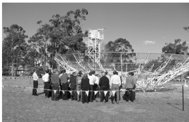
Figure 2: Participants at the "Antenna design for the xNTD" workshop admire one of the two 13.8-m diameter Fleurs telescope dishes, currently being refurbished on the Marsfield range. These antennas will form the NTD.
