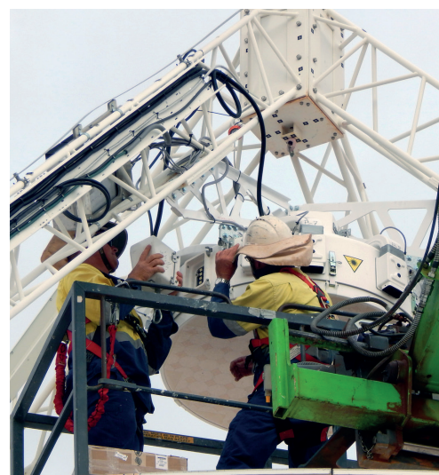
The Mk II prototype phased-array feed being installed onto ASKAP Antenna 29.
