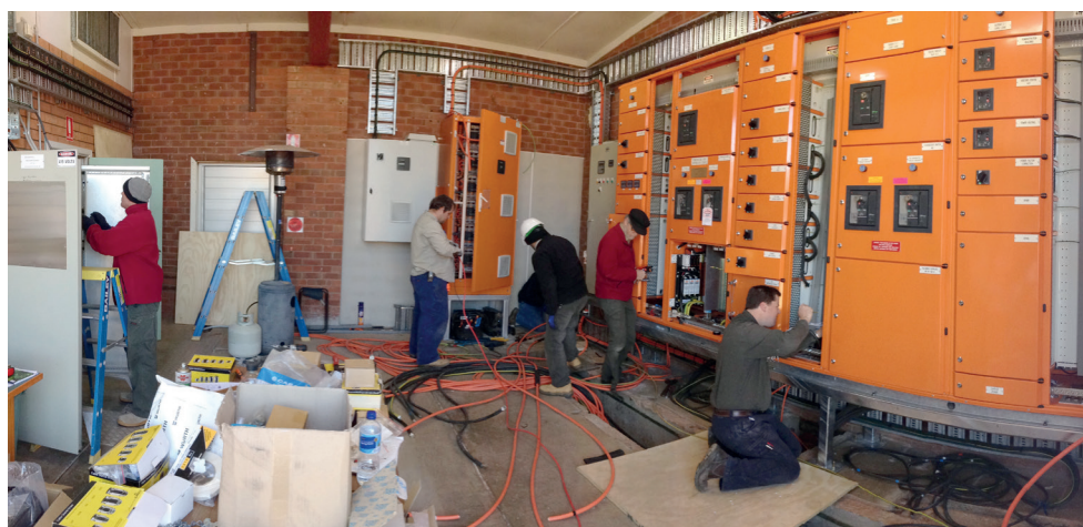
Installing the new electrical switchboard at Parkes
