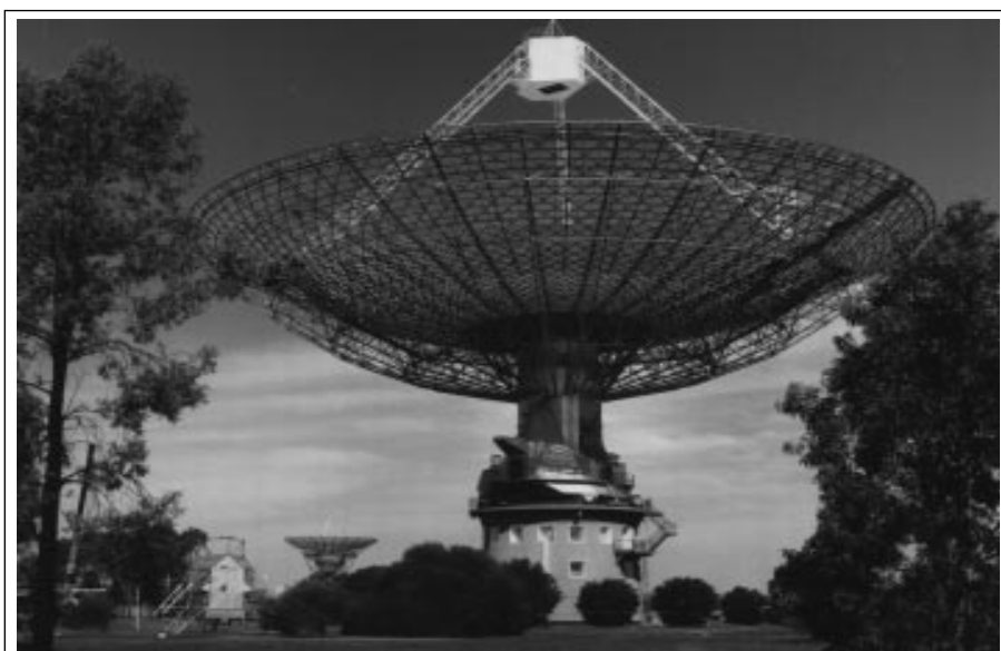
Parkes radio telescope with the new focus cabin.
