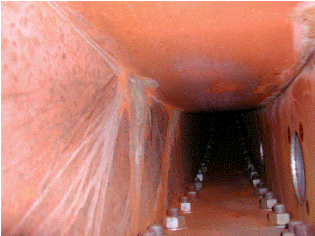
Fig 6: Signs of moisture ingress.
