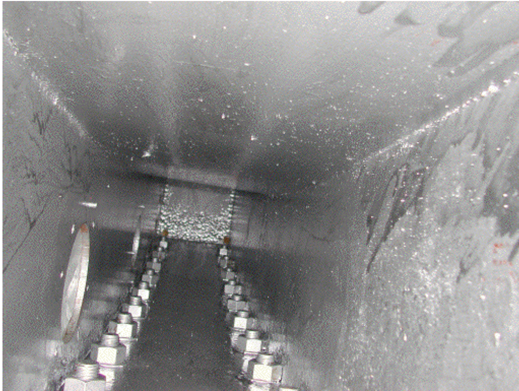
Fig 7: The finished job. Dark patches at the bottom are new drain holes.
