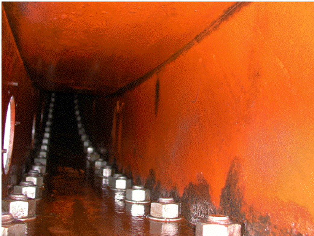
Fig 6: After rust converter application. Dark areas are neutralised rust.
