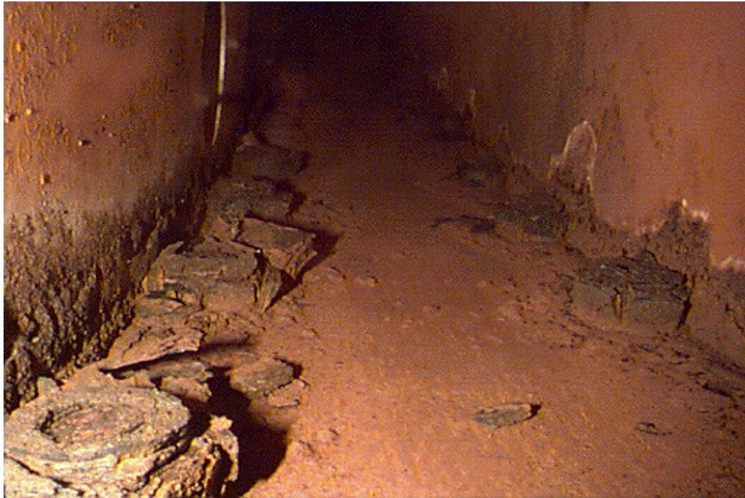
Fig 2: Corroded rack nuts and bolts inside the counterweight cavity.
