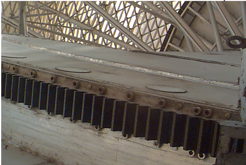
Fig 1: View of the right rack showing (face on) the rack teeth and bolt heads and (side on) the round access covers.
