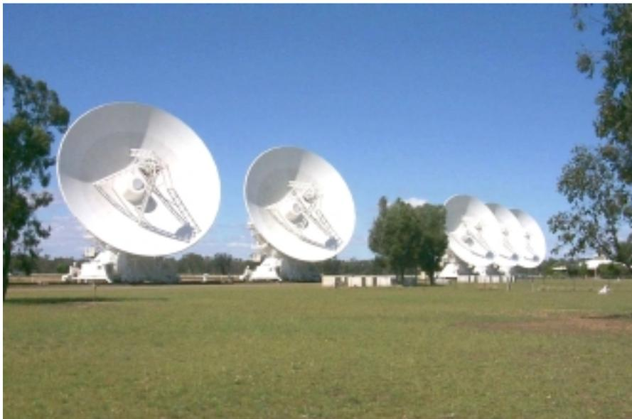
**Figure 4-3** Five antennas of the ATCA showing solid surfaces extending to the full diameter of 22 m
