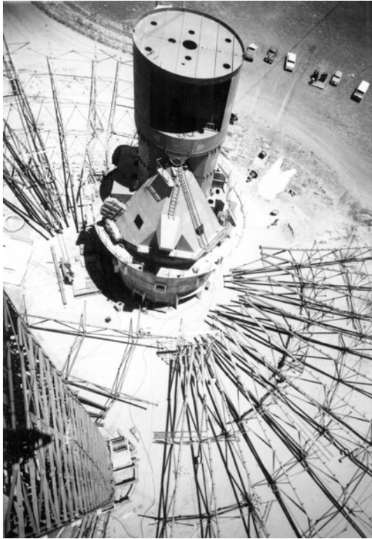
(left) The hub and pre-assembled rib sections. A thick layer of sand litters the site, used to sandblast the ribs prior to painting. (right) Lifting the first rib section into place. Each section was bolted to the hub and then to its neighbouring sections with a series of girders
