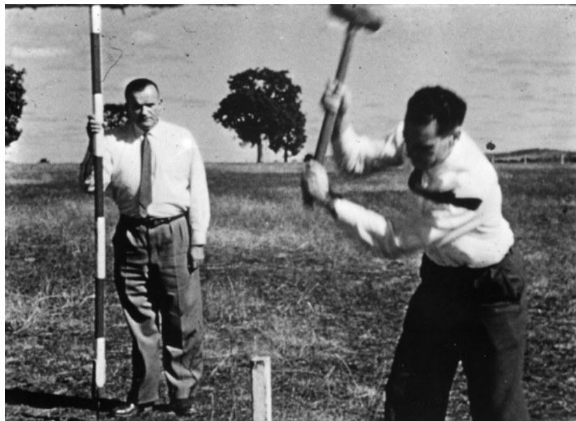
Taffy Bowen drives in a stake to mark the site of the telescope, while Lindsay McCready looks on. Well, not quite, it was a staged photo shoot. The real site was some distance away where earthworks had begun several weeks earlier. CSIRO bought the 170 hectare site – located about 20 km north of the Parkes township – from the sheep farmer Austie Helm
