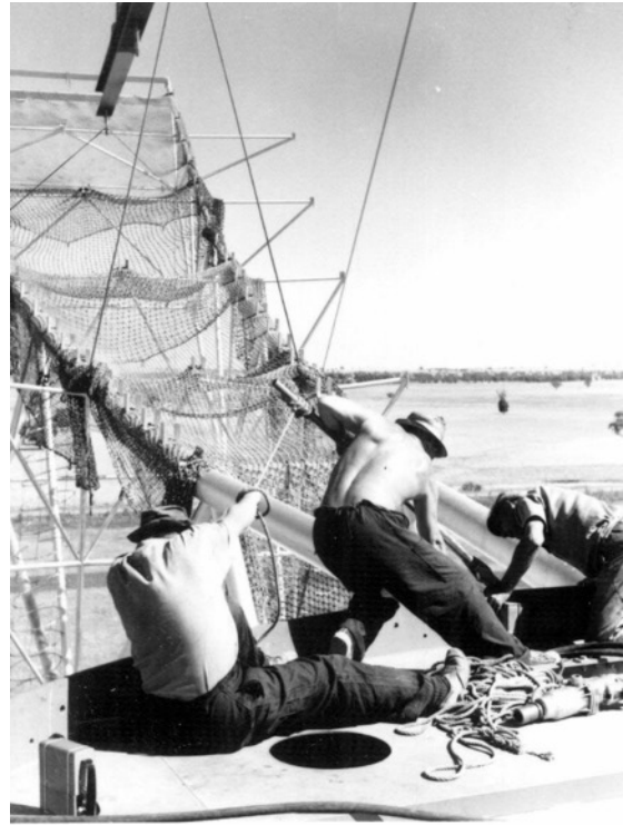
(left) The hub and pre-assembled rib sections. A thick layer of sand litters the site, used to sandblast the ribs prior to painting. (right) Lifting the first rib section into place. Each section was bolted to the hub and then to its neighbouring sections with a series of girders
