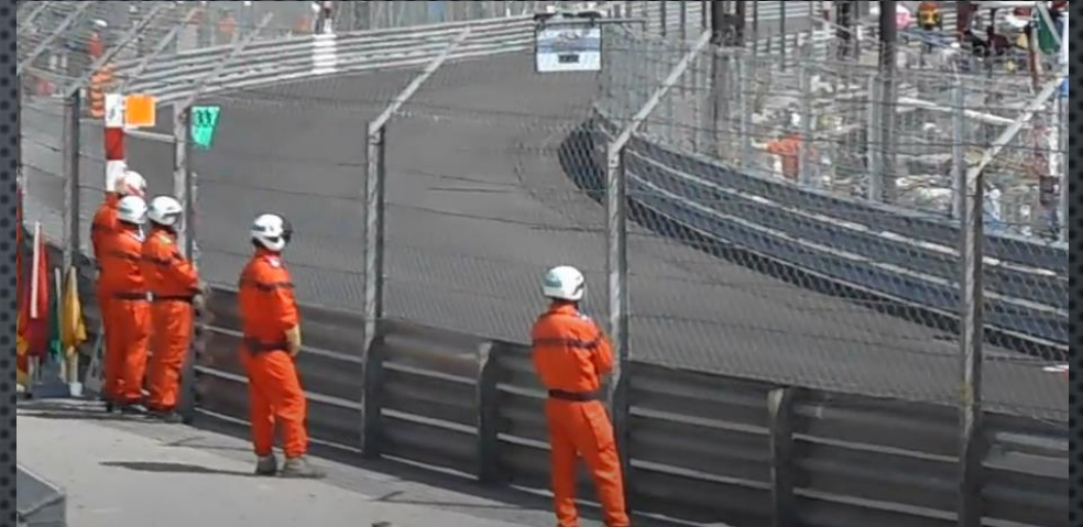
Armco Barrier (and Debris Fencing)
