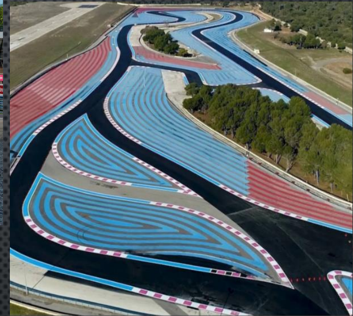
Circuit Paul-Ricard - Asphalt runoffs
