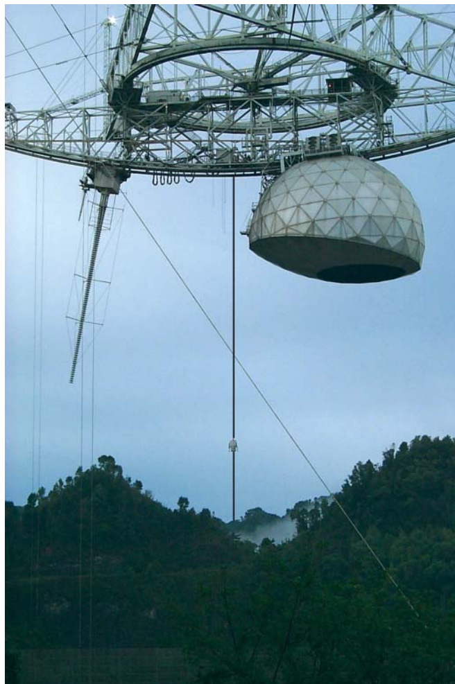
ALFA almost at its final destination, being lifted into the focus cabin of the Arecibo radio telescope. ALFA is the small object hanging above the background saddle.
