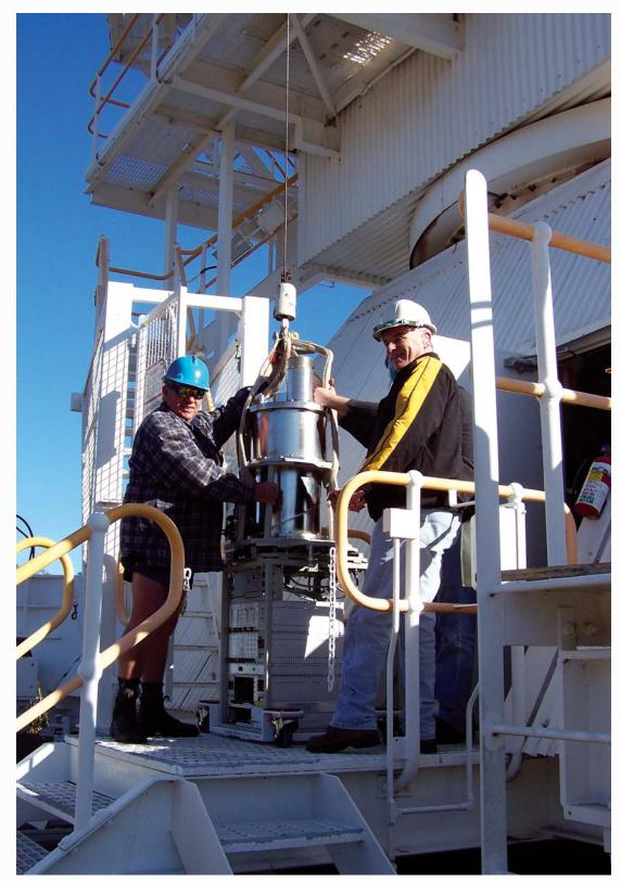
Bruce Tough (left) from Narrabri and Les Reilly (right) from Marsfield prepare the millimetre receiver, containing the prototype 7-mm components, for the lift to the turret and its final mounting position on antenna 6 of the Narrabri Compact Array.
