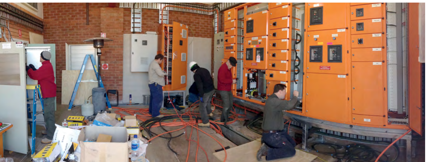
Installing the new electrical switchboard at Parkes
