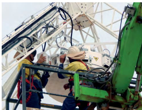
The prototype second-generation PAF going onto ASKAP Antenna 29.
