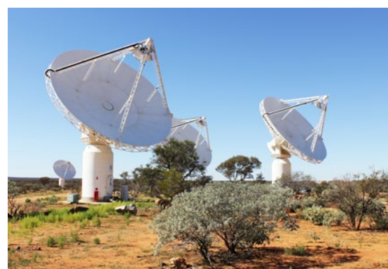
Antennas of the Australian SKA Pathfinder, ASKAP, at the Murchison Radio-astronomy Observatory in Western Australia. ASKAP began operating in 2014 with the first six of its 12-m antennas to be outfitted with CSIRO-developed phased-array feeds. Its final form the telescope will comprise 36 antennas. (Details, pages 34–35.) Credit: Flornes Yuen
