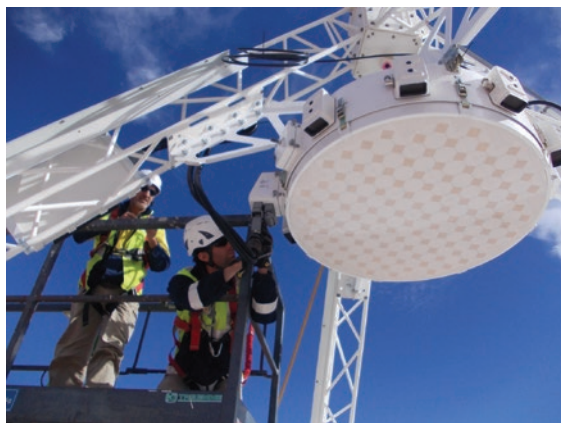
Installing a second-generation phased-array feed on an ASKAP antenna at the MRO Credit: CSIRO
