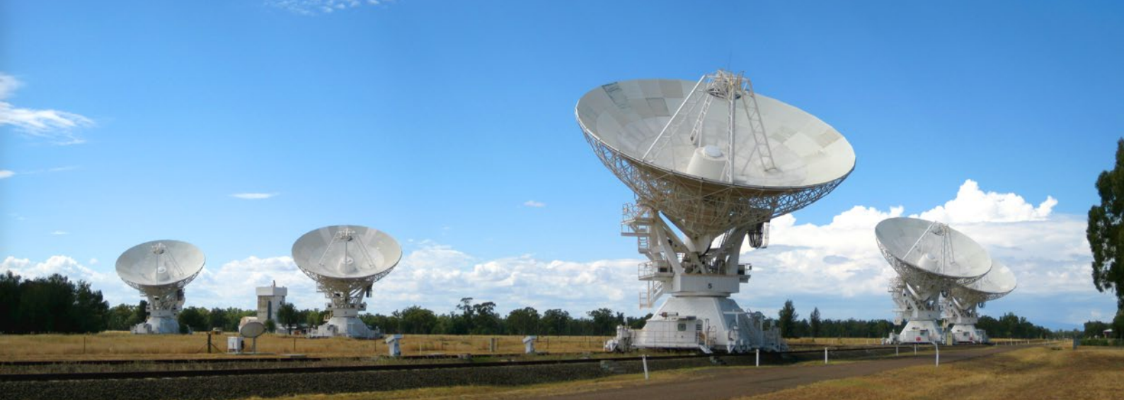
The Australia Telescope Compact Array, six 22-m diameter dishes near the town of Narrabri in New South Wales. The Compact Array can operate at frequencies between 1.0 GHz and 105 GHz, and its antennas ride on a six-kilometre track that allows multiple configurations and observing baselines. Credit: Cormac Purcell
