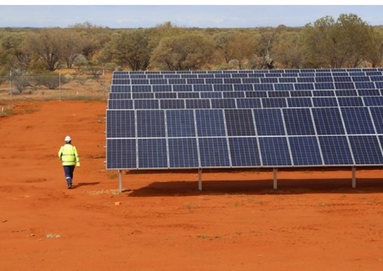
The solar array installed at the MRO in 2016 by Perth-based company Energy Made Clean (EMC). The array will be complemented by a 2.5 MWh battery system, and will supply a significant fraction of the observatory's power. Credit: Brett Hiscock
