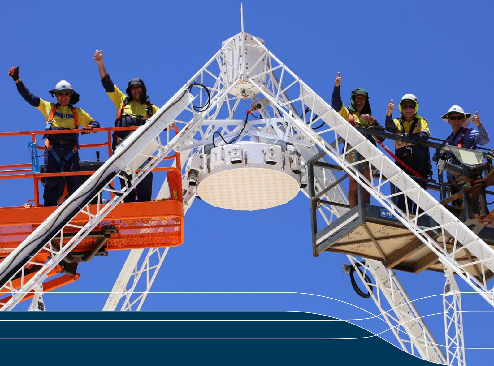
On 21 November 2017 the very last receiver was installed on ASKAP – meaning each of the 36 antennas now bears a second generation phased array feed. Image: Brett Hiscock.
