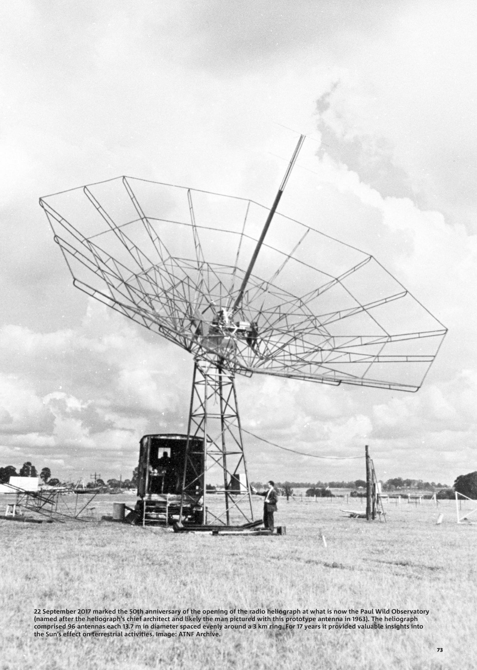
22 September 2017 marked the 50th anniversary of the opening of the radio heliograph at what is now the Paul Wild Observatory (named after the heliograph's chief architect and likely the man pictured with this prototype antenna in 1963). The heliograph comprised 96 antennas each 13.7 m in diameter spaced evenly around a 3 km ring. For 17 years it provided valuable insights into the Sun's effect on terrestrial activities. Image: ATNF Archive.
