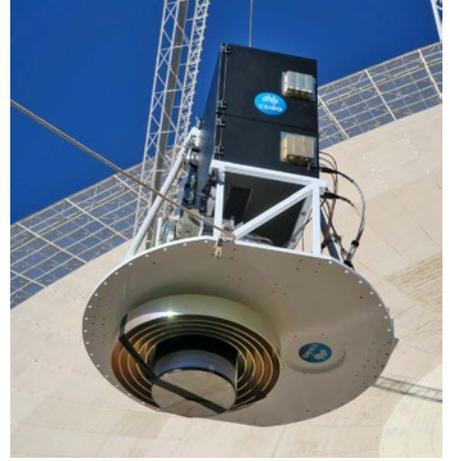
**The Ultra-Wideband Low receiver is hoisted into position on 15 May 2018. Image: John Sarkissian.**
