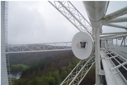
The PAF installed on the Effelsberg radio telescope in Germany. Image: MPIfR.
