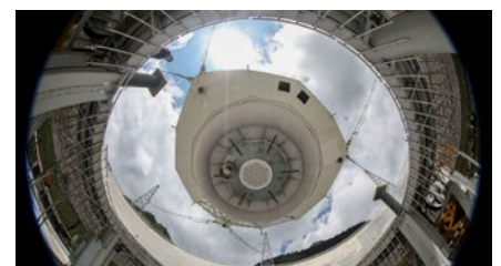
The focus cabin of FAST, with the 19-beam receiver on board, is hoisted into position. Image: Xinhua.
