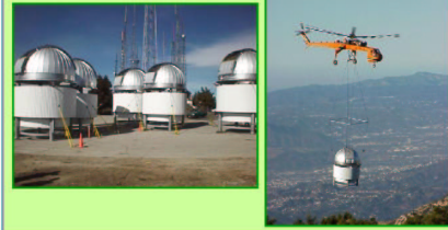
Telescope Enclosure Installation
