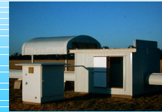
Siderostat Housing with Roll-off Roof
